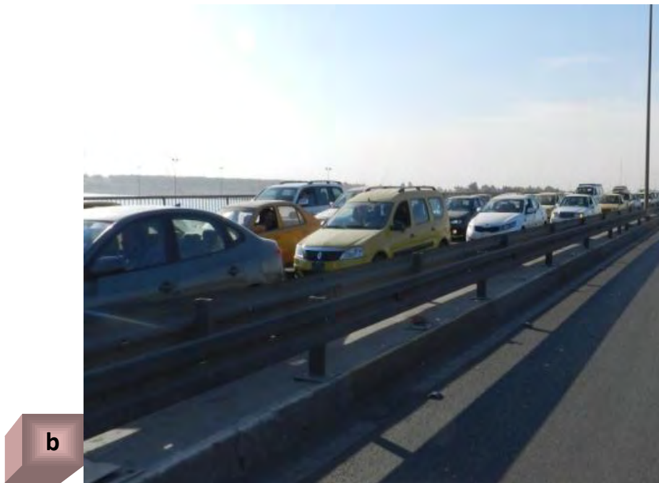
Figure. (13):a and b AL- Jadriah Bridge
