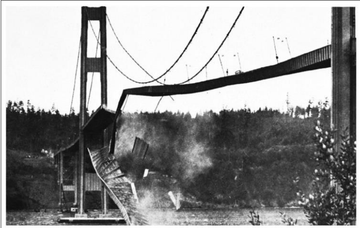
Fig.1 Tacoma Narrows bridge during wind-induced vibration. The bridge opened on July 1, 1940, and collapsed on November 7, 1940. (Farquharson photo, Historical Photography Collection, University of Washington Libraries-Rao).[6]
