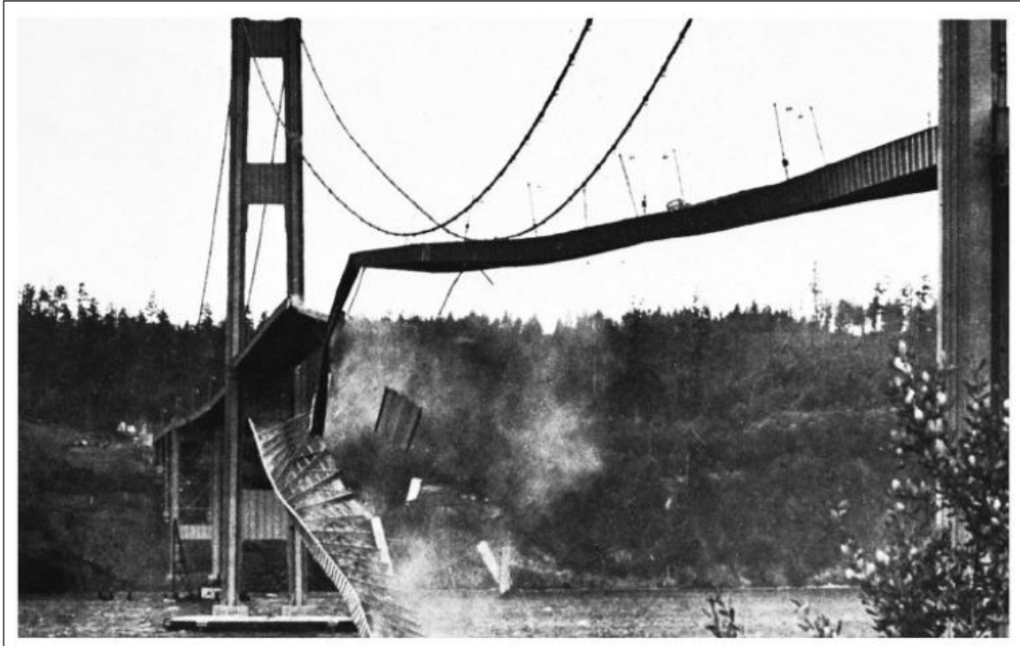
Fig.1 Tacoma Narrows bridge during wind-induced vibration. The bridge opened on July 1, 1940, and collapsed on November 7, 1940. (Farquharson photo, Historical Photography Collection, University of Washington Libraries-Rao).[6]
